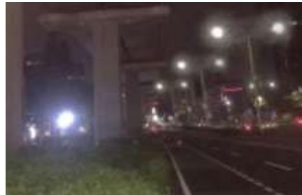
Figure 7 Addition of lighting lamps
