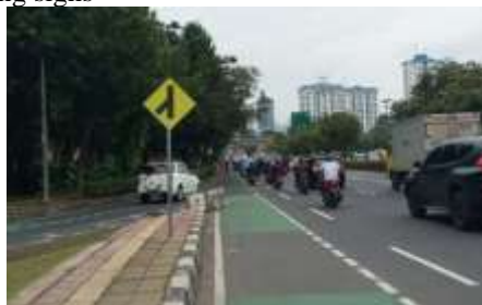
Figure 9 Installation of warning signs
