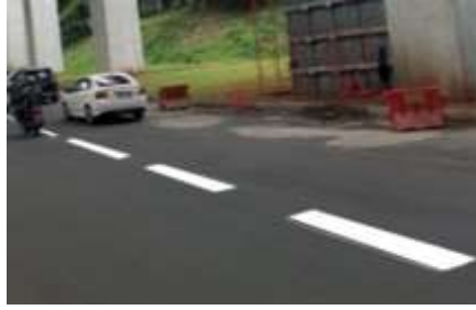
Figure 6 Road markings creation
