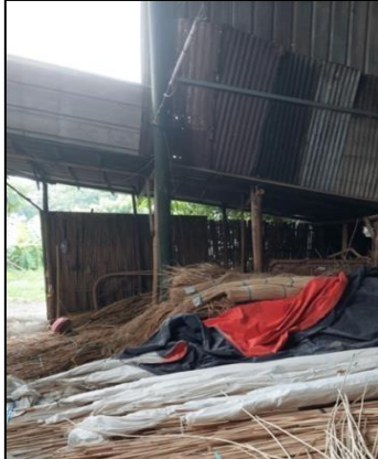
Figure 11. Condition before being covered with a tarpaulin
