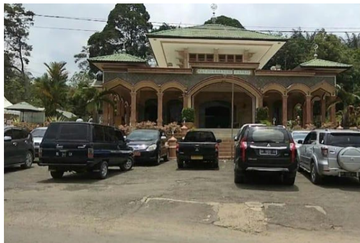
Figure 3. Parking Area in Front of Babur Rahmat Mosque
