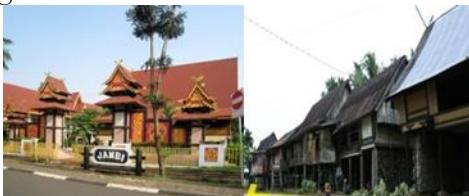
Figure 7. Simple roof shapes and ornaments of the Jambi Malay community style that are traditionally made on a human scale
